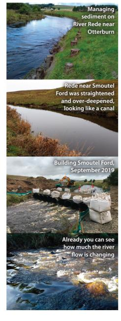
cut the eroding bank to form a shallower angle of slope, set the new fencing further back into the field, and secured seeded coir matting to help hold the soil in place. These changes will now allow the river to move across the floodplain and keep grazing animals off the bank edges.
