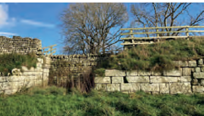
The West gate. On the left are the mounded cap and springer, which supported the arch. Towers built of large stone blocks were on either side.
